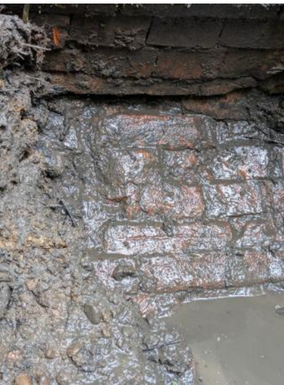
mains of the old culvert that took the Spondon Bourne under the canal. The team report
