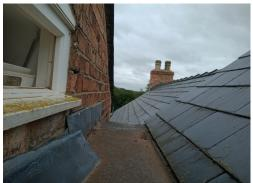
At the cottages we have discovered a leak in the flashing around a roof valley and it's been repaired very quickly.
