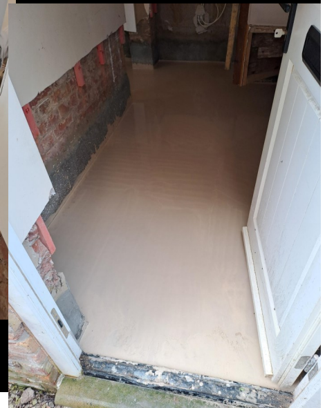
New screed laid
